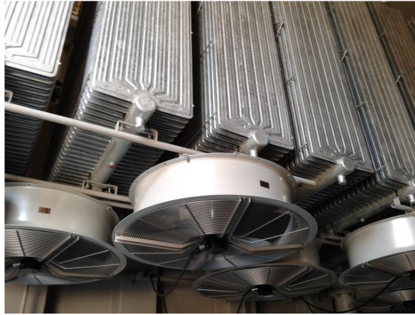
Figure 1: Axial fans mounted for vertical airflow on oil-cooled transformers. Source: ebm-papst Inc.
